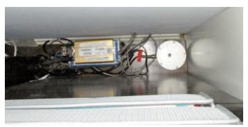
Figure 4. Looking down at typical vibration monitor installation.
