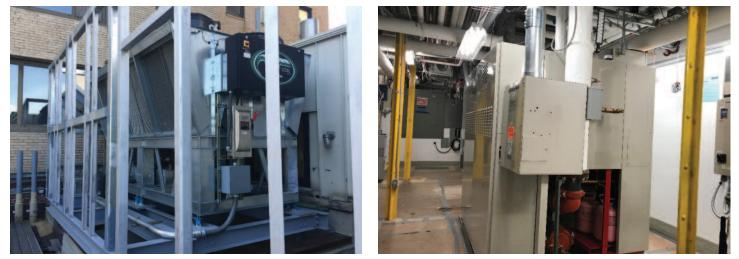
Figure 7. Completed chiller installation: from roof (left) and in new fifth-floor mechanical room (right).
