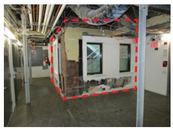
Figure 3. Interior view of load-bearing masonry walls to be removed on fifth floor.
