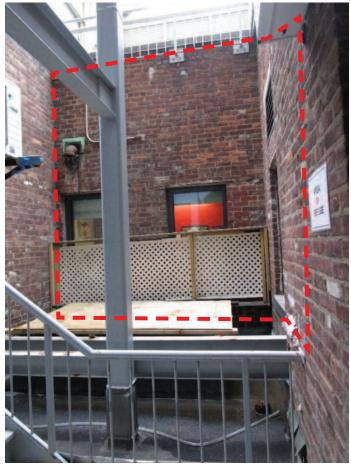
Figure 2. Brick masonry removal area at fifth floor, adjacent to new chiller location.
